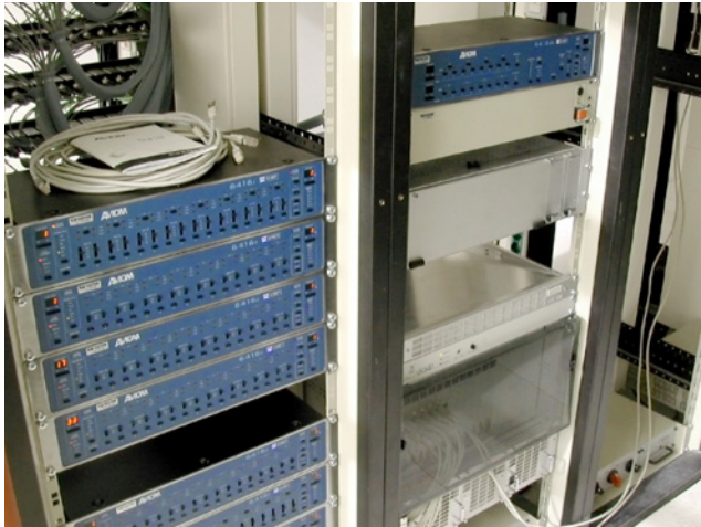
Pro64 Input and Output Modules at Videotime Studios
